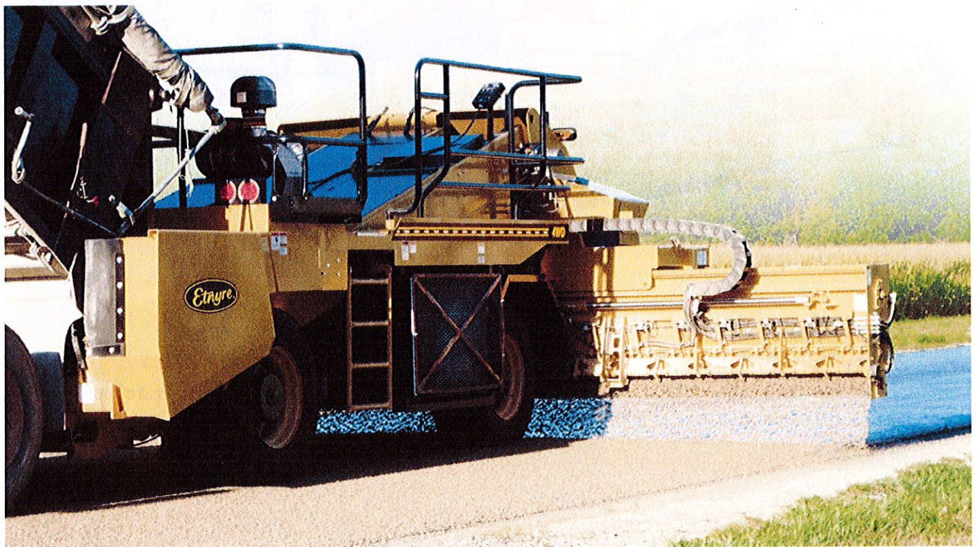
ChipSpreader with four wheel drive and variable width spread hopper
