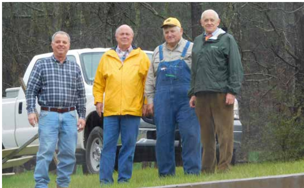
Inspecting a culvert on County Road 59 during the Randolph County DRIVE-Along Tour. From left, County Engineer Burrell Jones, Rep. Bob Fincher, Commissioner Terry Lovvorn and Sen. Gerald Dial.
